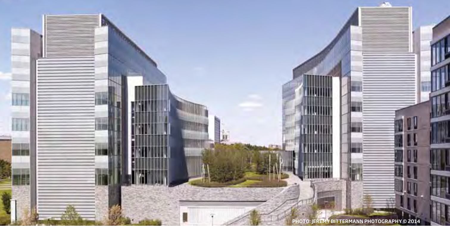
Aerial view of CUNY Advanced Science Research Center & CCNY Center for Discovery and Innovation in Harlem
