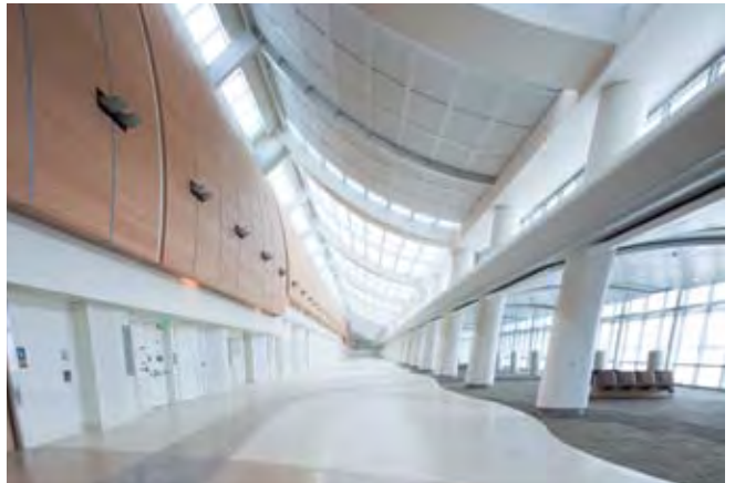
Norman Y. Mineta San Jose International Airport Capital Improvement Project, San Jose, CA, the third largest airport in California and on track to achieve LEED-Silver certification. Architect: Gensler and Associates
