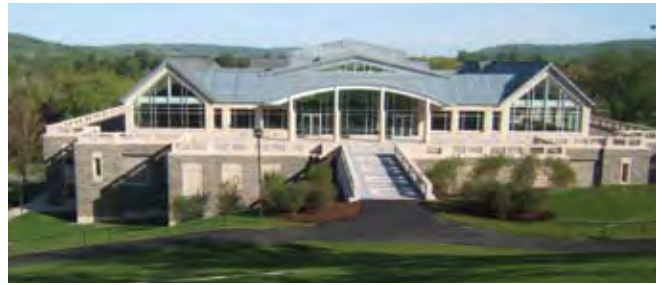
Case Library Center for Information Technology, Colgate University, Hamilton, NY. Architect: Shepley Bulfinch Richardson Abbott
