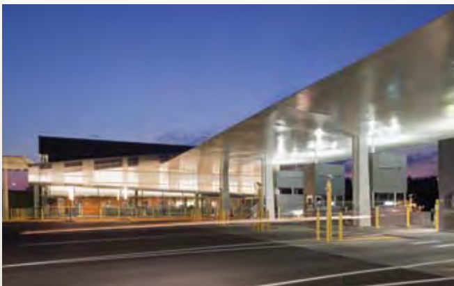
U.S. Land Port of Entry, General Services Administration, Massena, NY, LEED NC-Silver Certification. Architect: Smith-Miller & Hawkinson (SM+H)
