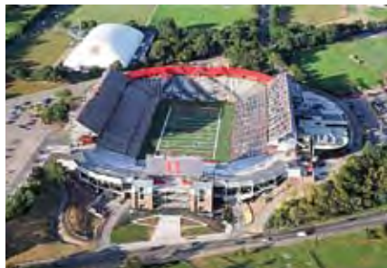
Rutgers University Football Stadium Expansion, Piscataway, NJ. Architect: Populous (Fmr. HOK Sport)
