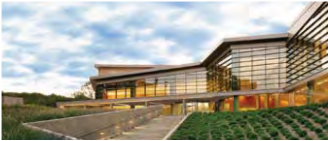
Stony Brook Medical Center, State University of New York (SUNY), Stony Brook, NY. Architect: Cannon Design
